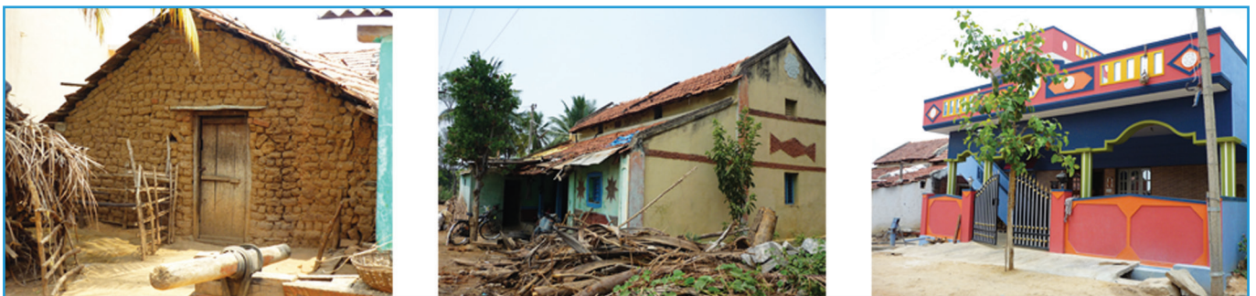
Figure 4 A sample of building types in Ungra village: gabled roof adobe house (left), gabled roof brick plastered house with verandah (centre), and flat roof concrete dwelling with compound wall and parking space (right)
