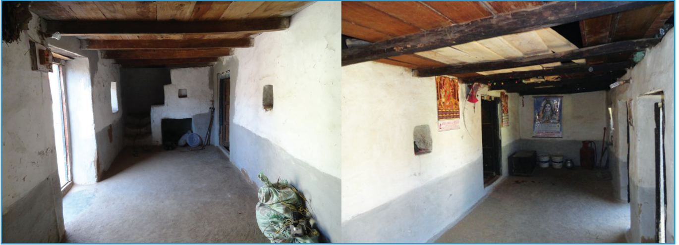
Figure 4 View of ground and top floor of selected traditional house in Mandi, Himachal Pradesh
