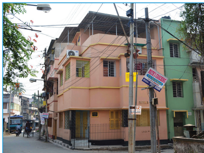
Figure 2 A two storey building with AC on top floor and GI-shed over roof
