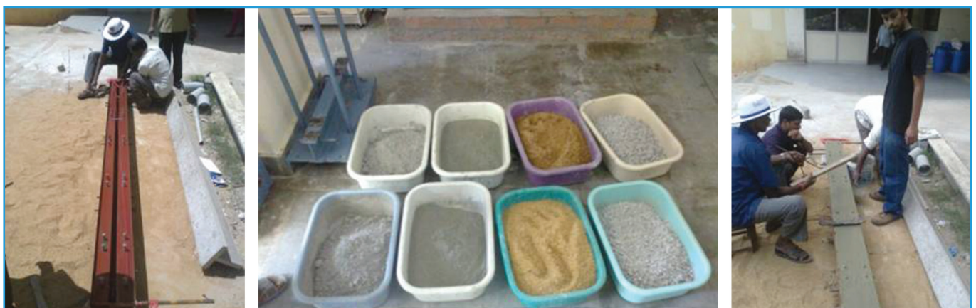
Preparation of reinforcement
