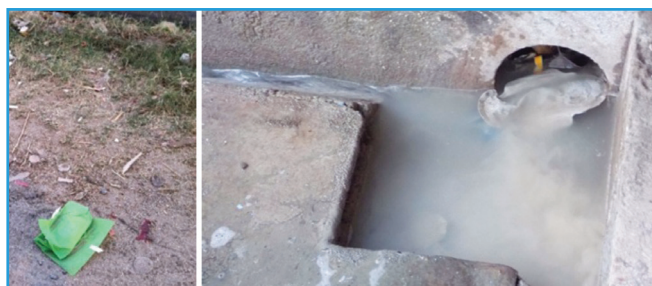
Figure 7 Sanitary napkin packet thrown by the wayside and a napkin choking a water outlet
