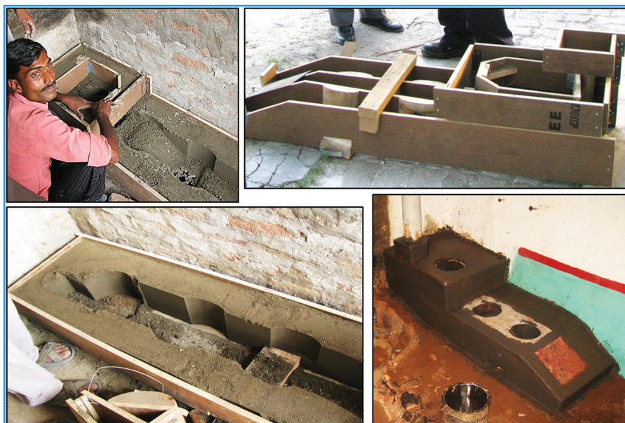
Figure 6 Using the mould to construct Astra ole
