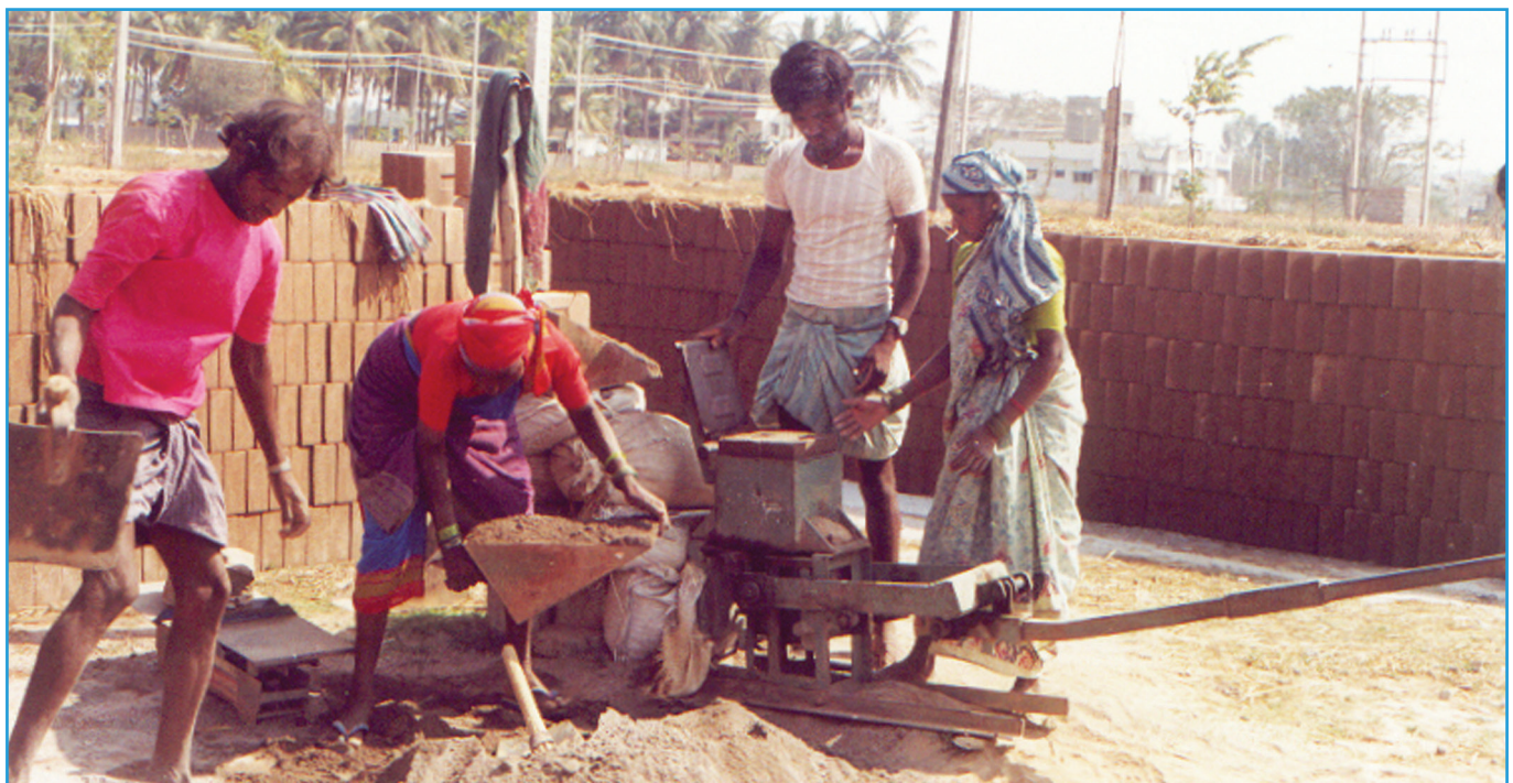
Figure 8 Block making in progress at a construction site
