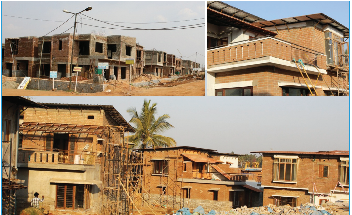
Figure 14 Cluster of SSB masonry houses in the case study project (Bangalore, India)
