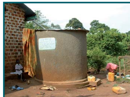
Water harvested into the container (Tank) through gutters
