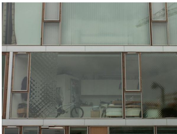
Fig. 9 The same system applied to a conventional glass facade could help control transparency as well as internal climate.
