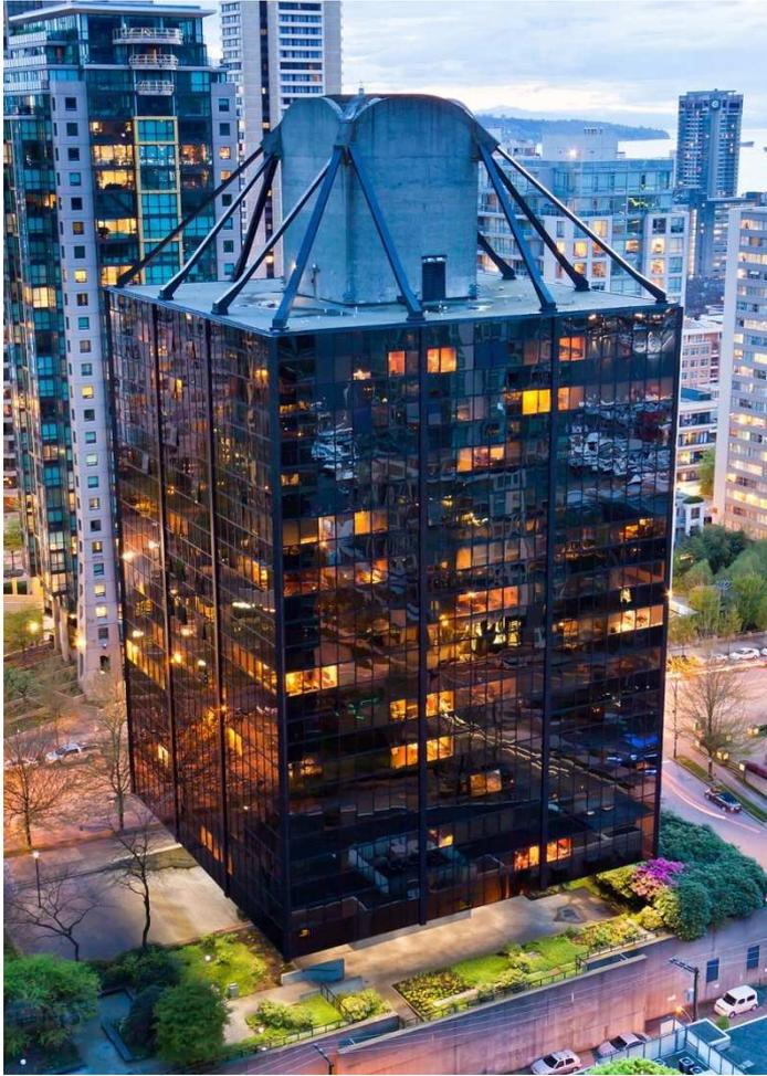
**Figure 29 The Qube, Vancouver.** Architects in Canada agreed on it being one of the most earthquake-proof buildings there (Vancouver Sun, 2004), though unfortunately no analysis has been published. The impressive concrete core is decisive for seismic proofing, and could likely be combined with illumination elements in future buildings with a similar building plan. Taken from Abirkill, Wikimedia Commons.
